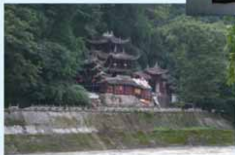
国家重点文物保护单位二王庙古建筑群留真毁假 The original foundations of Erwang Temple, were almost unaffected, while the imitation of ancient buildings were damaged.
